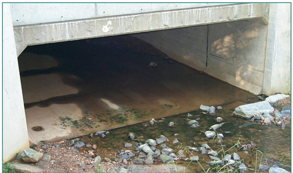
Wide, shallow flow prevents fish from moving freely upstream and downstream.
